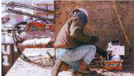
The PE60 used for pre-stressing.
